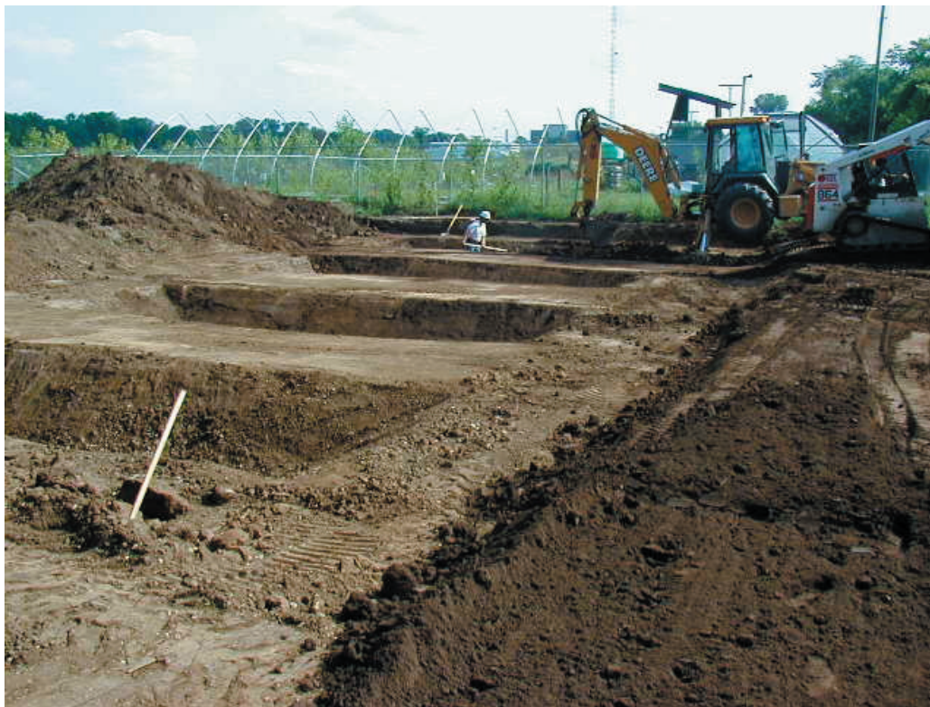
Figure 5. Excavation of wetland basins, August 30, 2000
