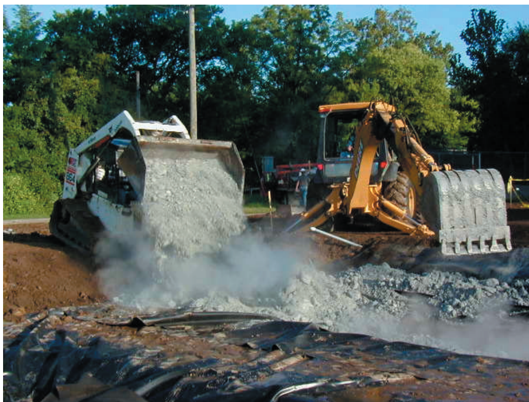
Figure 7. Addition of FGD material to two experimental wetland basins, September 13, 2000
