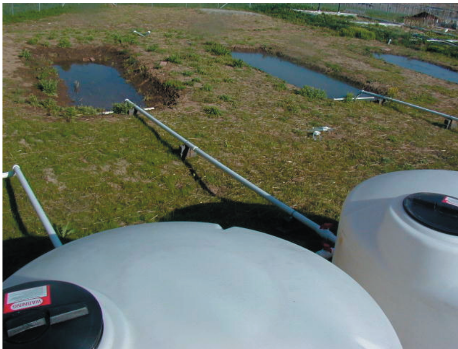
Figure 9. Installation of water delivery system to experimental wetland basins, April 25, 2001
