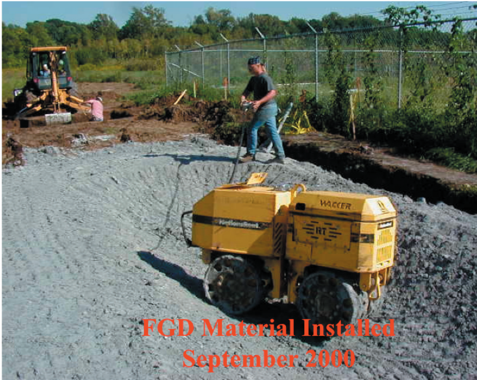
Figure 8. Liner in FGD wetland basin showing initial compaction, September 13, 2000
