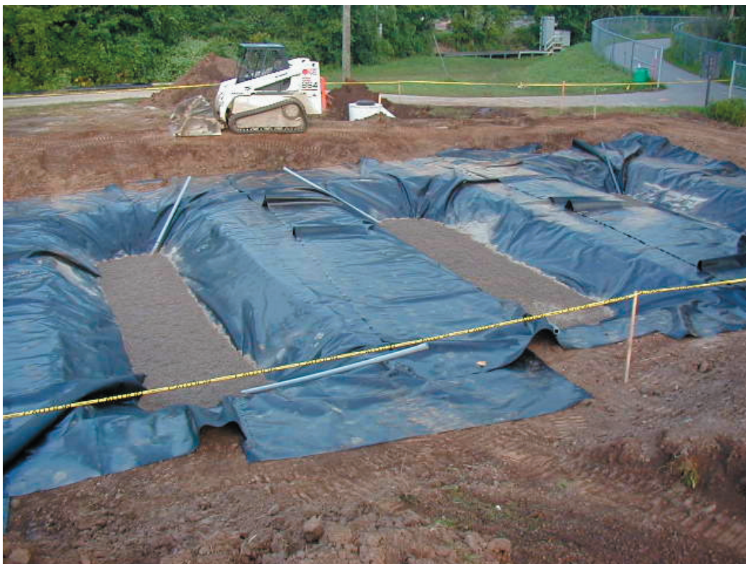
Figure 6. Placement of impervious liners and leachate collection system, September 1, 2000
