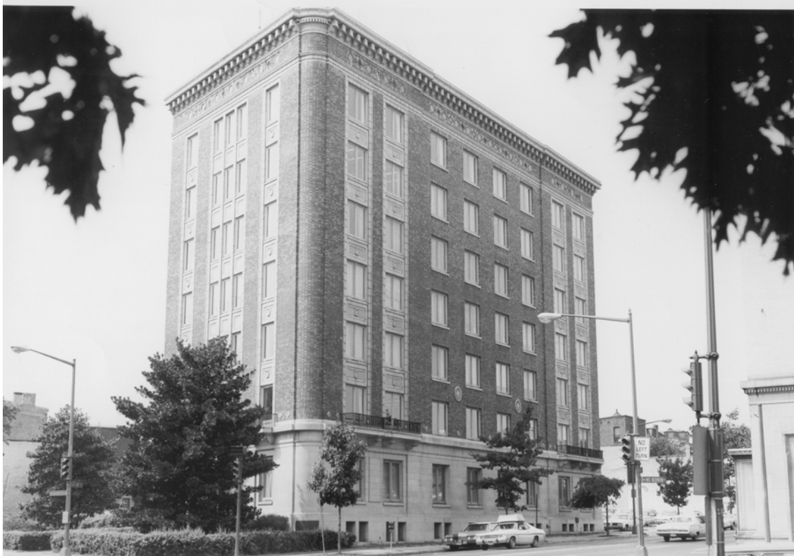
American Federation of Labor Building National Park Service
