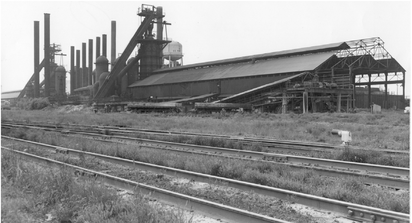
Sloss Furnace Photo by Bill Wilson Studio
