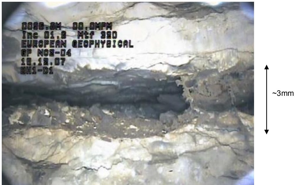
Figure 9-5 CCTV survey, potential fracture at 84mbgl – borehole 1
