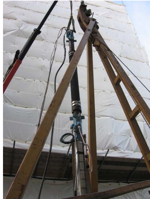
Figure 4. Equipment being lowered into the borehole
