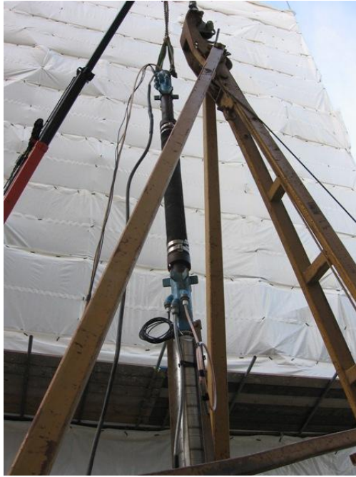
Figure 9-11 Equipment being lowered into the borehole
