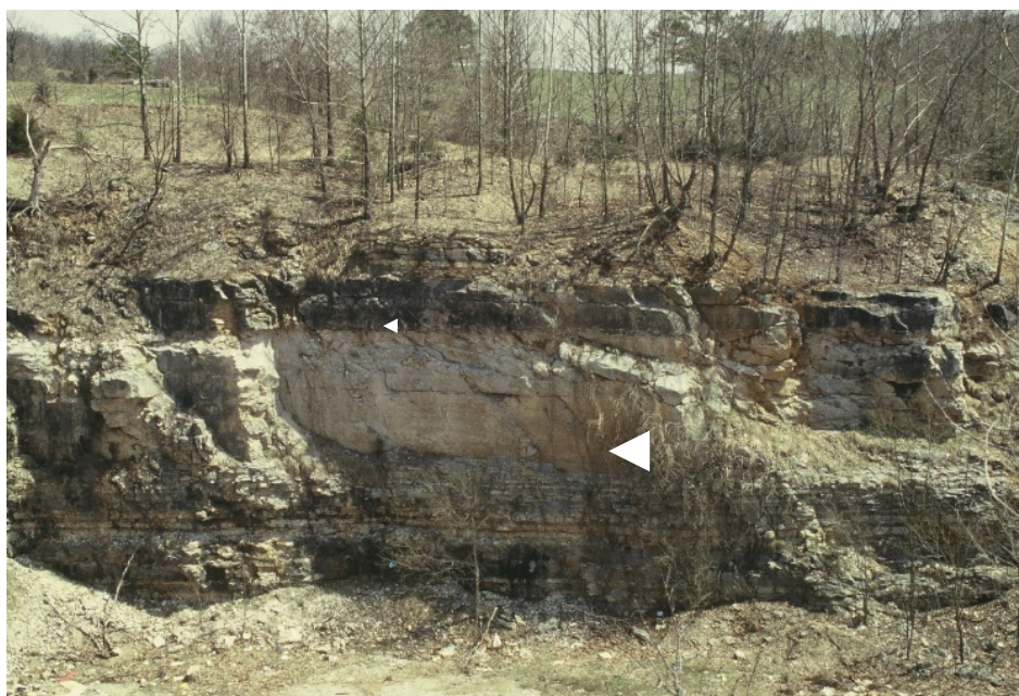
Fig. 1. Short Creek Oolite exposed in the abandoned War Eagle Quarry, on the south side of U.S. Highway 412, accessible on a road just east of the bridge over War Eagle Creek between Old Alabam and Harmony, Madison County, Arkansas. Upper Boone exhibits sharp, planar contacts above and below a 7.6 m (25 ft) interval of Short Creek Oolite (white arrows). This locality was studied by Lisle (1983).
