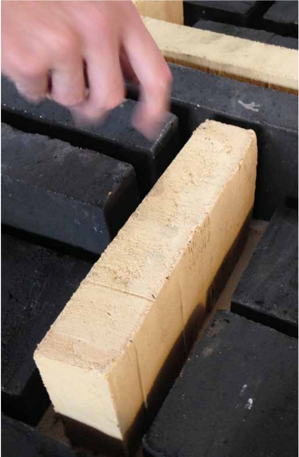
Figure 1: Brickwork bond combining two similar bricks but with different colours into a thermally composite heterogeneous masonry structure. Photo by author.
