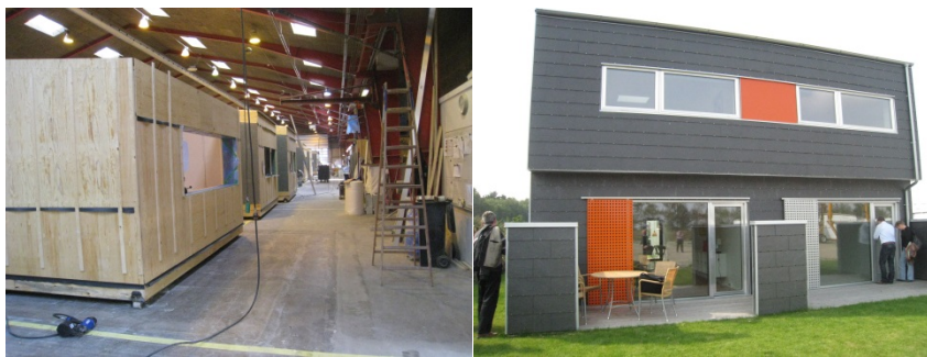
Figure 1. The housing units in SH+ are based on design concepts in frameworks (bundled tenders), allowing indoor prefab production with a large number of housing units (left picture, from the producer ScandiByg, who won the Framework 1 with 525 housing units). For the buyers, small variations are allowed within the general design, e.g. the type of materials on the façade, the size of the flats etc. For this purpose, a 1:1 test-house has been built at the production facility in Løgstør (right picture).
