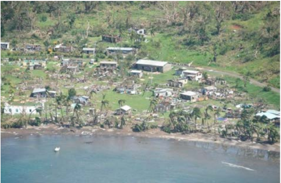
Fiji. Damage of cyclone Winston, February 2016. Source: EMPICS.
