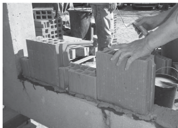
Figure 3. Construction of masonry wall.
