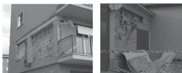
Figure 2. Detachment of the leaves in multi leaf walls (Braga et al., 2011).
