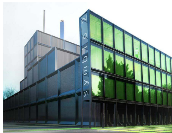
Fig. 12. Waste incineration processing plant with 300 m 2 biofacade PBR in Nantes.
