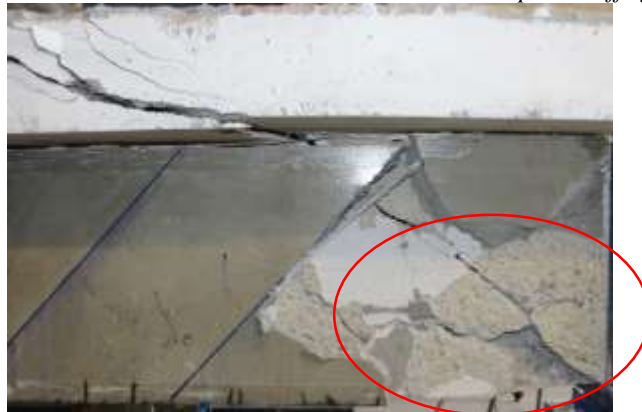
c) Local detachment of HCPs at failure load
