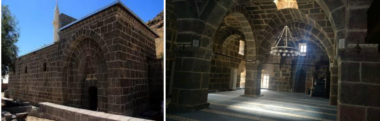
Figure 2: Outside and inside of the Elti Hatun Mosque
