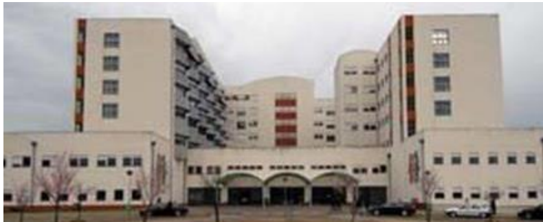
Figure 3 – General view of Building B.
