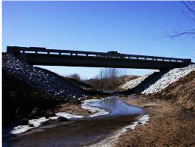
Figure 2.6: Mars Hill Bridge, Iowa, Canada.
