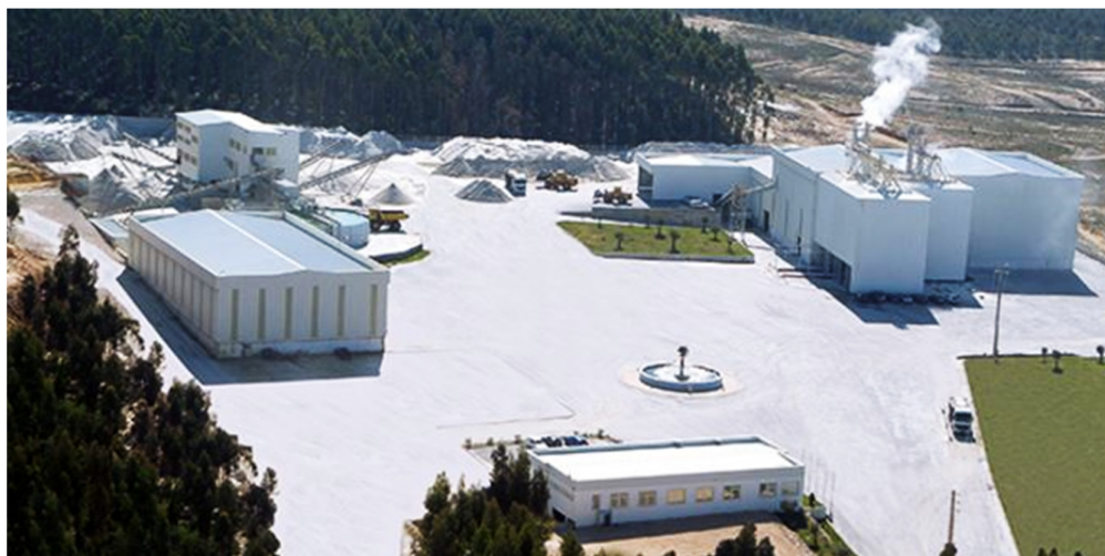
Figure 3.3: Parapedra Group job site situated in Rio Mior, Portugal ( http://www.parapedra.pt/en/sifucel.php ).
