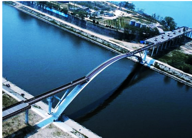
Figure 2.5: Sunyudo (Peace) Footbridge on Han River in Seoul (Ductal®, 2002).
