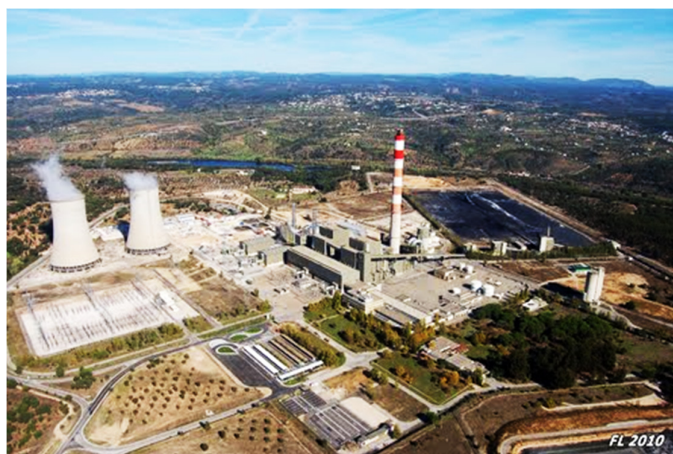
Figure 3.1: A view of Pego power station (Lopes, 2010).
