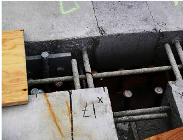
Figure 2.7: Joints between precast panels and shear connector panels, Rainy Lake, Ontario.
