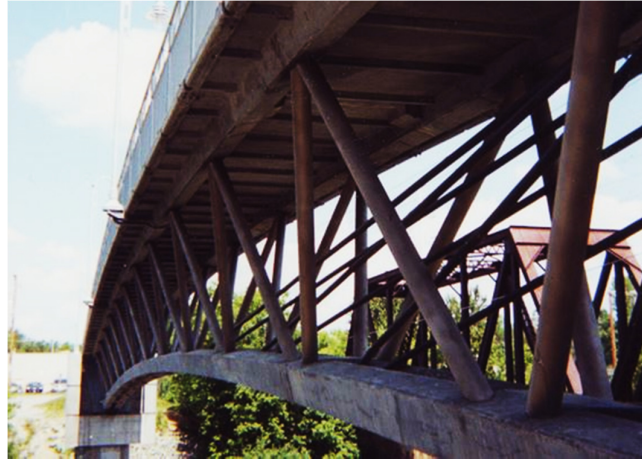
Figure 2.4: Sherbrooke Pedestrian Overpass, Canada (Ductal®, 1997).
