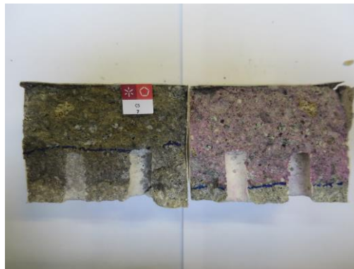
Figure 3: Chloride depth (left) and Carbonation depth (right) reached in group A.
