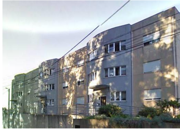
Figure 1 - Main façade of the building.
