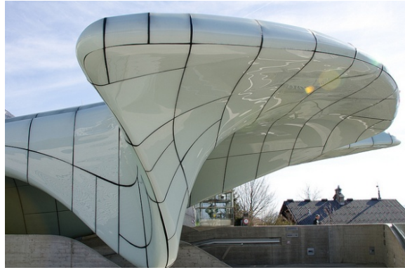
Figure 1: Hungerburg funicular station (Austria) Project: Zara Hadid Architects Available in: www.flickr.com
