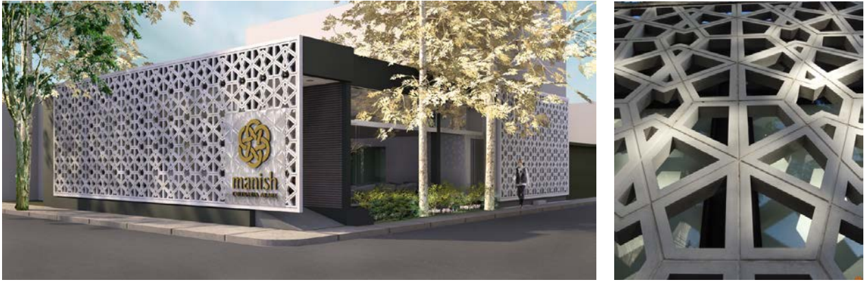
Figure 4: Arabic restaurant in São Paulo. Project: ODVO Architecture and Urbanism. Courtesy: Wincret Designer Concrete Products.
