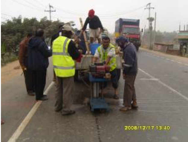
Plate 7.13 (b): Coring of Bituminous layer has in progress at N4 road
