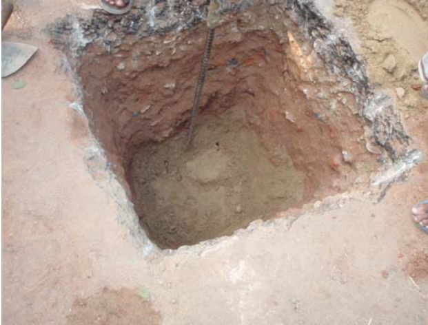
Plate 7.9: Digging of trail pits manually
