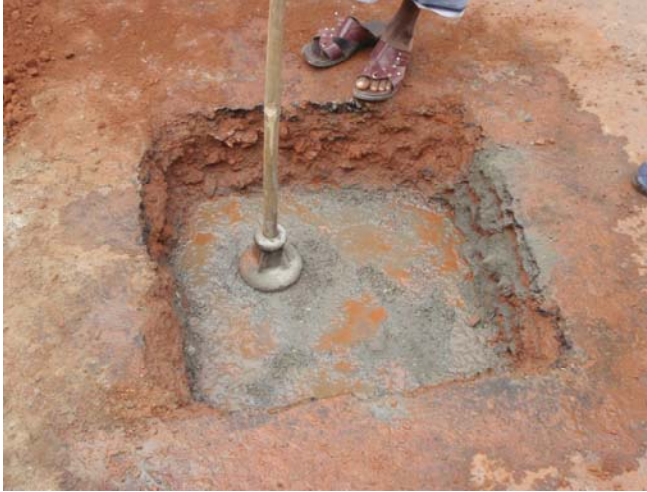
Plate 7.11: Reinstatement of granular layer of trial pits using aggregate + 5% cement.
