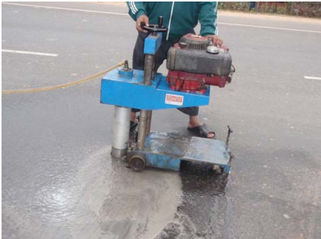
Plate 7.13 (a): Coring of Bituminous layer has in progress at N4 road
