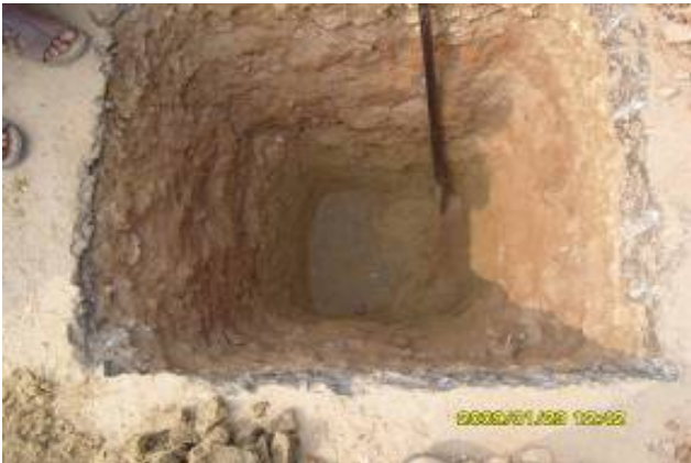
Plate 7.10: Trail Pit at N4 road (Old bituminous layer below ISG)
