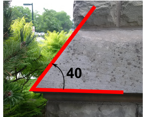
Figure 5.4: A close-up image of the inclination of surface 6. The upward normal from the horizontal is the \Gamma_\alpha recorded. In this case, the angle is 40^\circ
