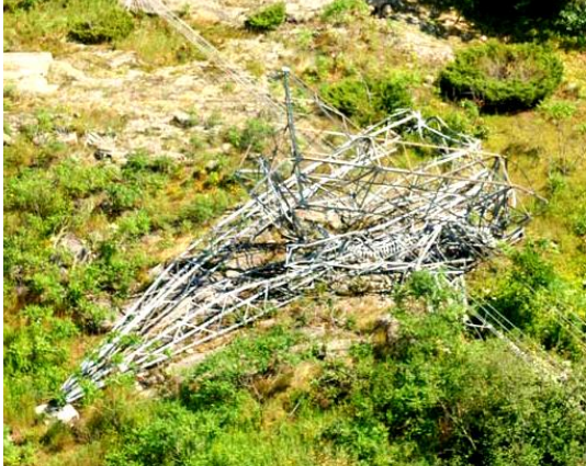
Fig. 2-1. Guyed tower failure in Ontario, (Hydro One Report, 2006).
