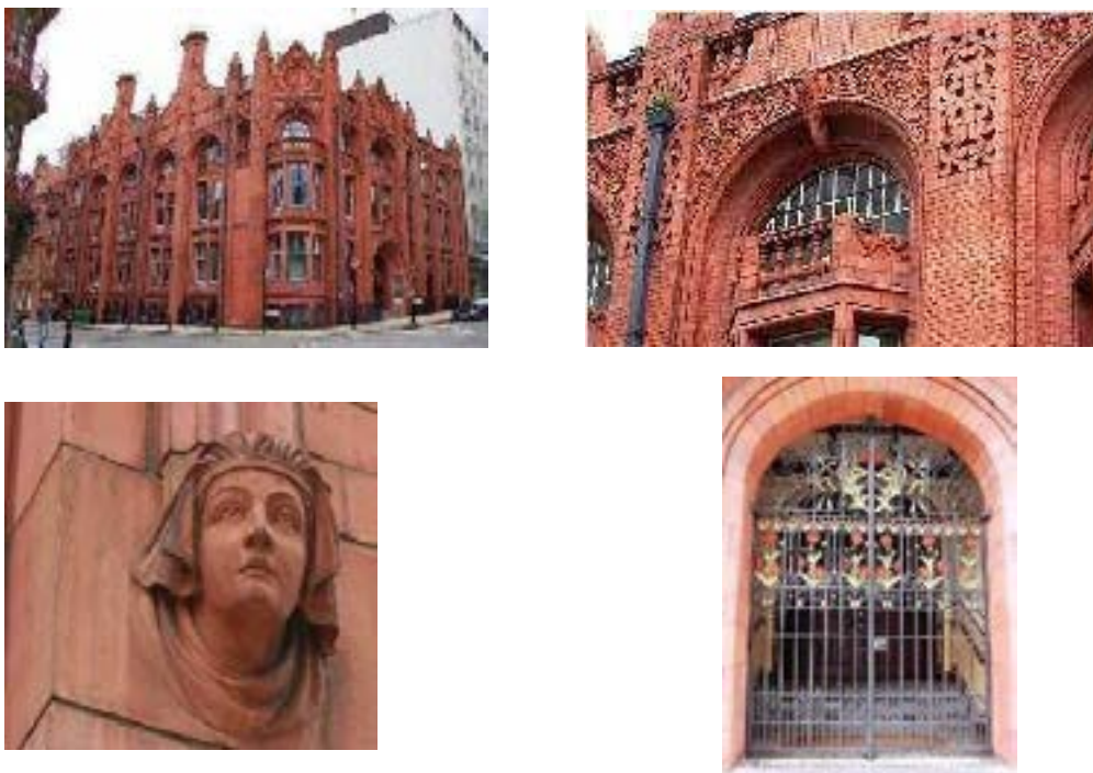
Figura 78: National Telephone Company , Birmingham (Reino Unido), 1896, Frederick Martin. Vista general y detalles. Fotografías: James "Buildingfan" (Flickr).
