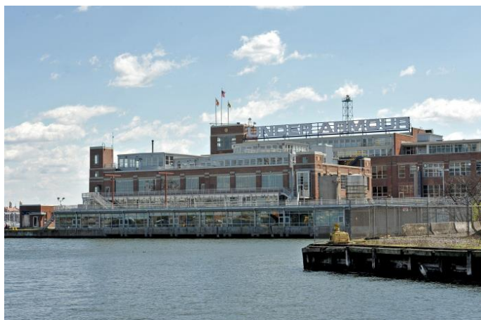
Figure 12-UA headquarters in Baltimore (source: The Columbus Dispatch)
