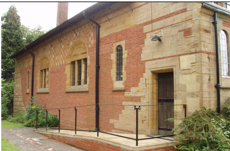
Figs 27- 29. Details of the patterned stone and brickwork on the exterior of the Church of the Wisdom of God.
