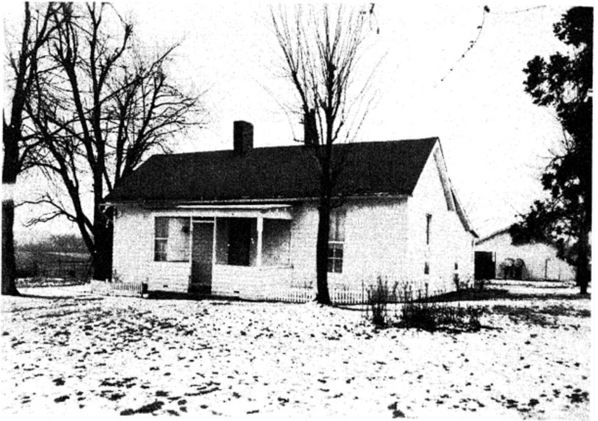
Figure 9. Test House No. 3 as seen from the northwest corner.
