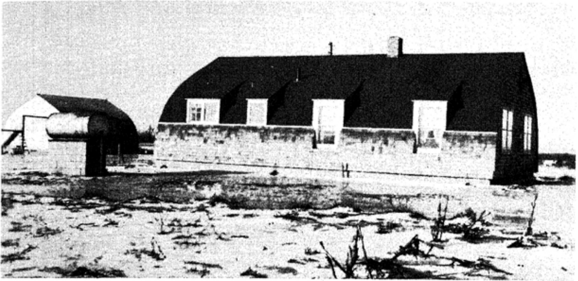
Figure 6. Test House No. 2 as seen from the northeast corner.
