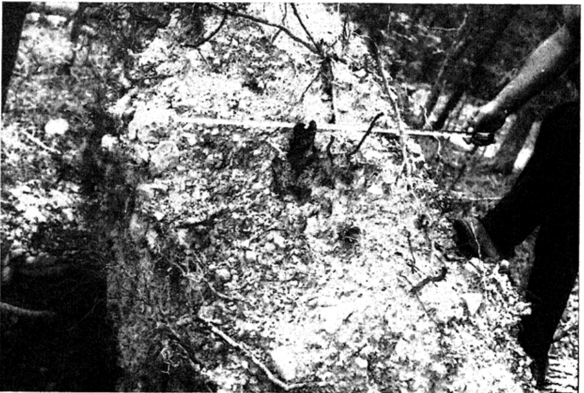
U.S. FOREST SERVICE PHOTO N.O. 10,063. Flat bottom of soil mass exposed by wind-thrown 18-inch white oak. Zone occupied by roots is about 25-30 inches thick, and most feeding roots are in upper half of soil mass. Tree grew in mid position on moderate slope in southeastern Shannon County.
