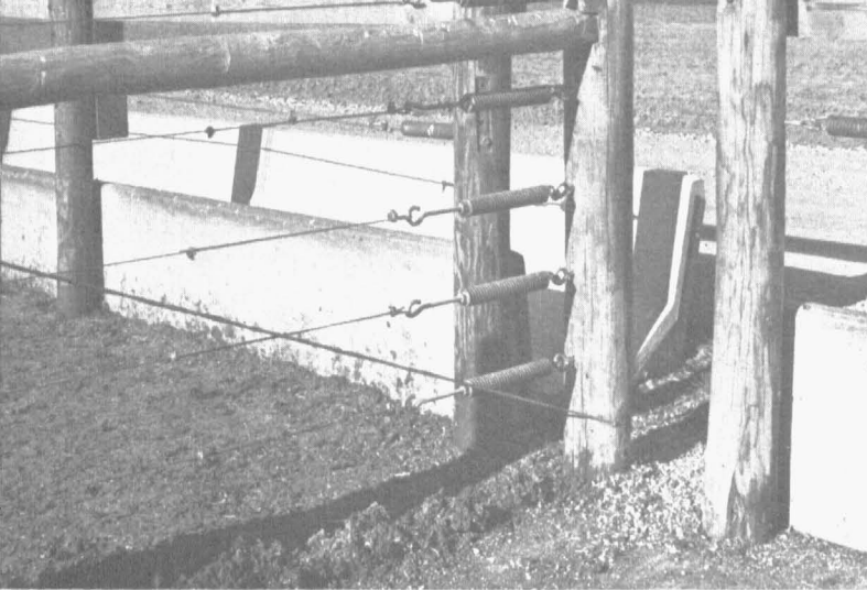
Spring loaded cables make good dividing fences. Six strands would be better; some animals got through this five-strand fence.
