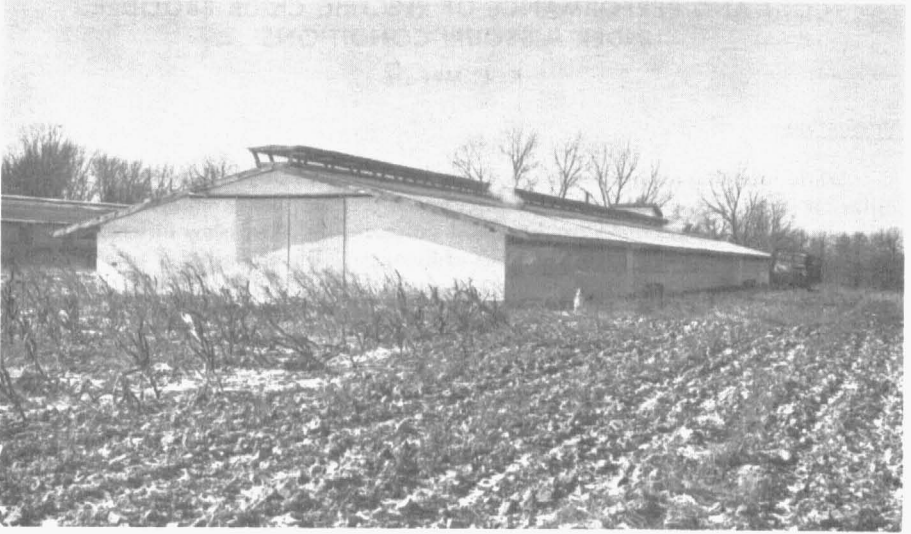
Fig. 1—The uninsulated 40' x 200' frame house, equipped with a ridge vent and 4 mil plastic curtain windows.
