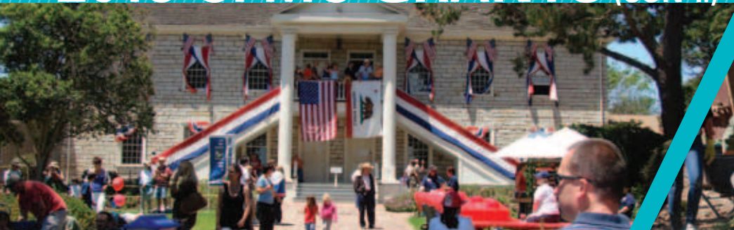
▶ Historic preservation grantee Colton Hall decked out for the 4th of July
