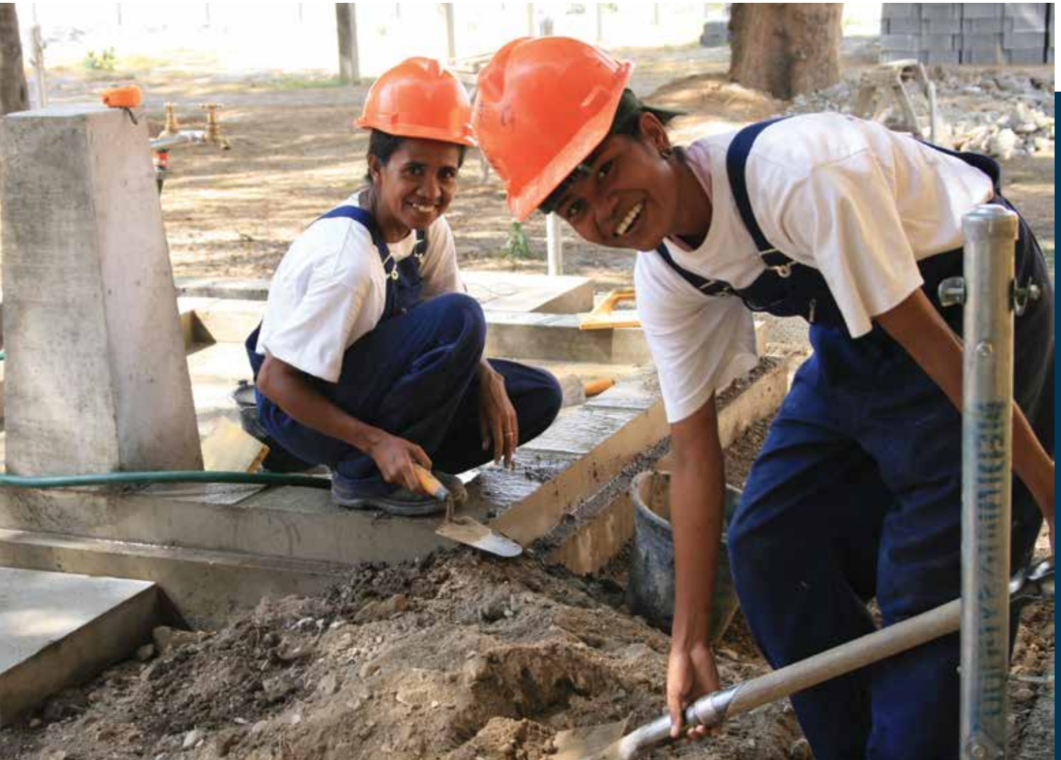
Training for women plumbers (Timor Leste) Photo: © AusAID
