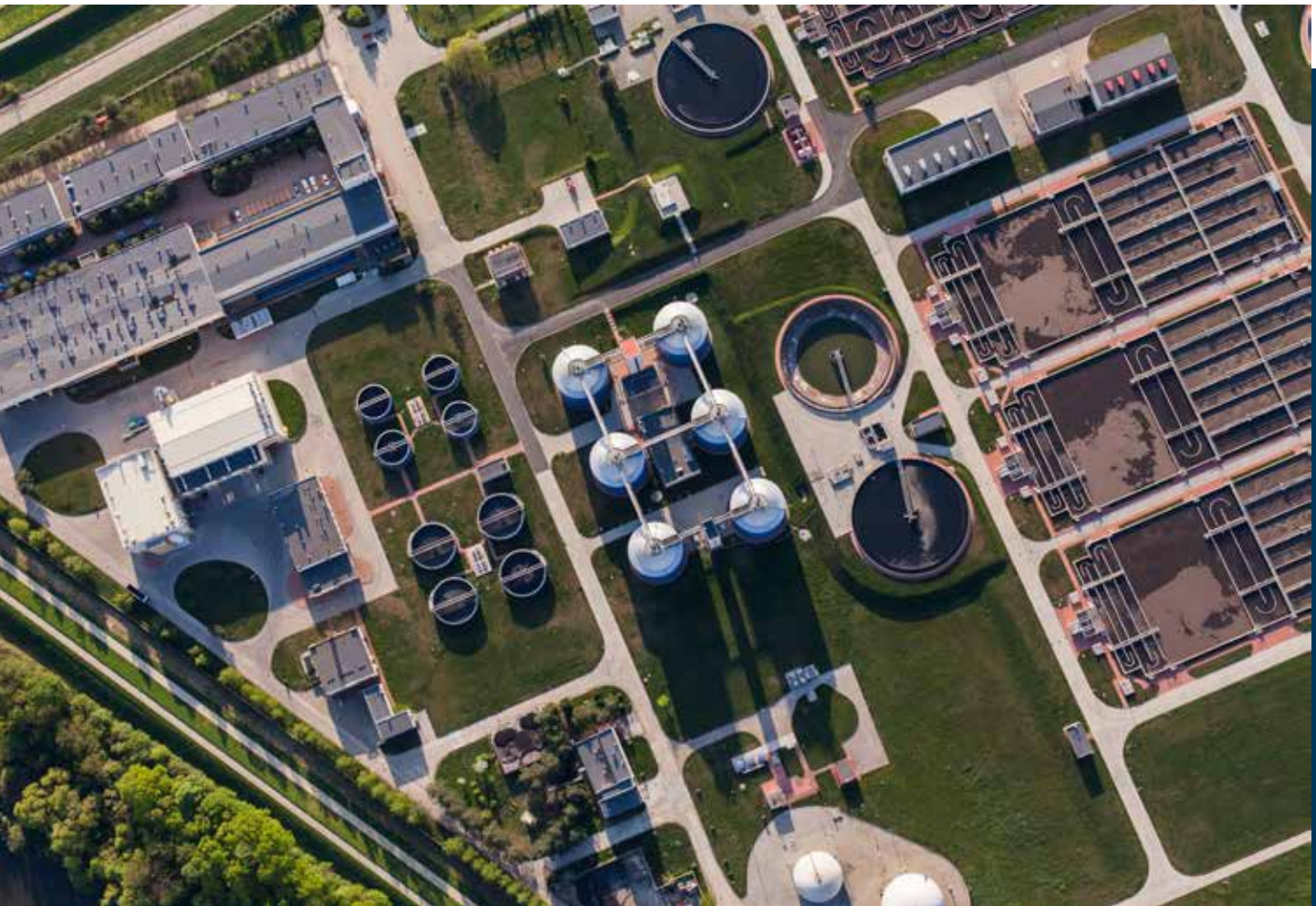
Aerial view of a sewage treatment plant Photo: © iStock.com/Mariusz Szczygiel
