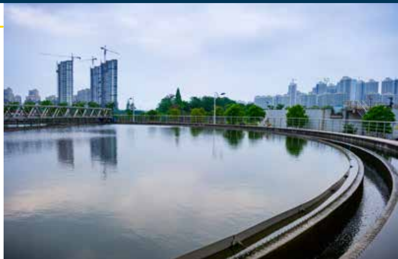
Modern urban wastewater treatment plant Photo: © hxdyl/Shutterstock.com
