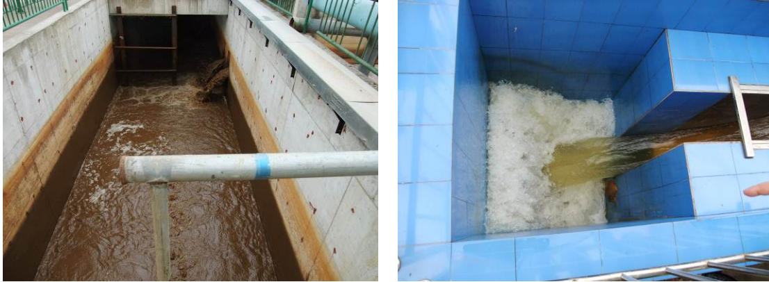
Figure 1. In Shangsi County, water from a sugar plant is treated before it is mixed with river water and used for irrigation. The photo on the left shows untreated water and the photo on the right shows treated water.
