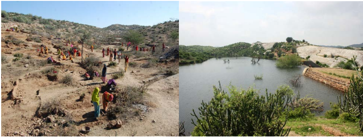
Check dam (before and after construction) at Paluna village in Rajasthan
