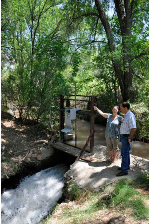
New Automated Headgate Diversion Structure
