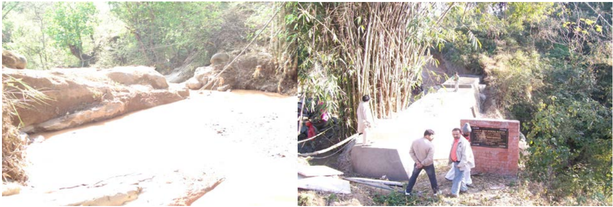
Check dam (before and after construction) at Bedu Khuua village in Himachal Pradesh
