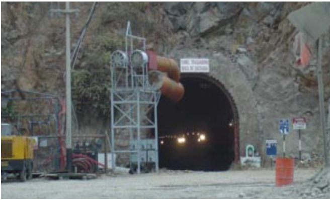
Photo 6: Start Trans Andes Tunnel © Credit: WWF / W.Nagel
