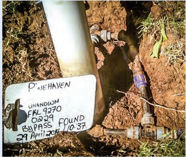
Tampering (left) and bypassing (right) have fallen sharply in Mogale City since the municipality appointed a service provider to do regular visual monitoring, meter reading, and exception reporting.
