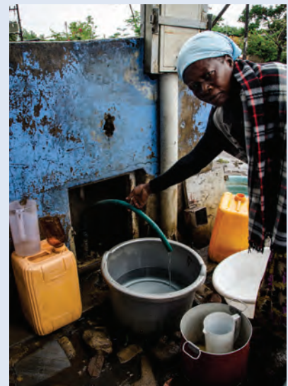
Bypassed prepaid standpipe meters because of low water pressure in Kanyama, Lusaka. The utility has now installed a conventional meter and tap ahead of each prepaid standpipe, and tap attendants sell the water per container for cash, bypassing the disabled prepaid device.
