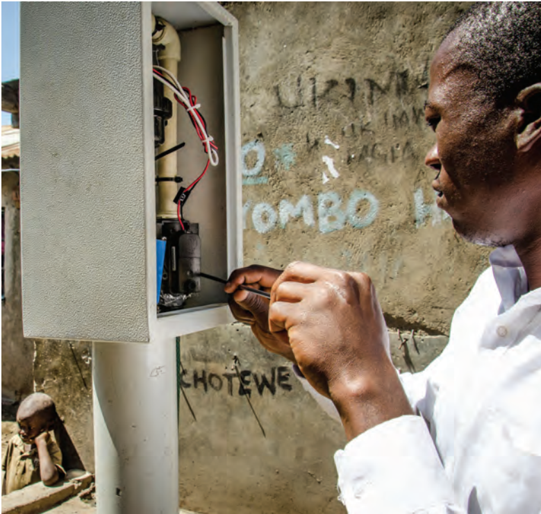
FIGURE 16: COLLINS OUMA, A SELF-TAUGHT METER REPAIRMAN IN NAKURU, KENYA, REPAIRS A LEAKING SEAL WITH A MAKESHIFT PLASTIC GASKET
