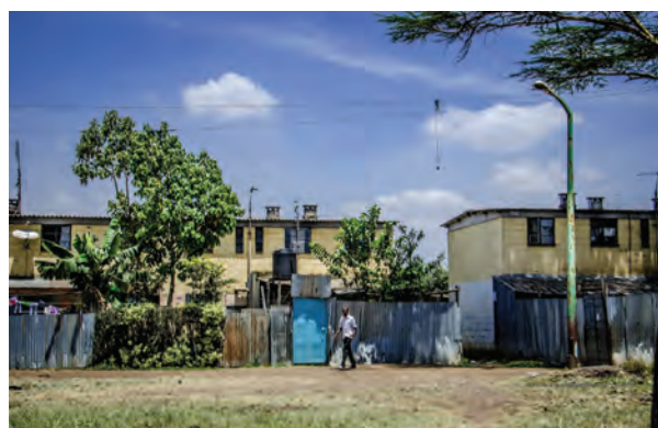
FIGURE 7: PREPAID METERS HAVE BEEN IN USE IN JERICHO, A LOW-INCOME COUNCIL HOUSING ESTATE IN NAIROBI, SINCE 2011
