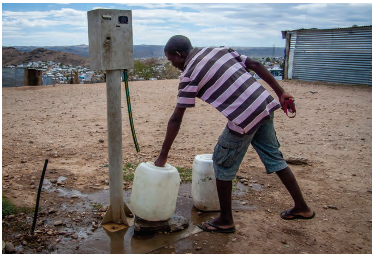
FIGURE 3: A PREPAID METER ON A SHARED PUBLIC STAND POST
