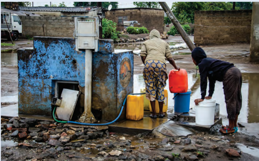
Bypassed prepaid standpipe meters because of low water pressure in Kanyama, Lusaka. The utility has now installed a conventional meter and tap ahead of each prepaid standpipe, and tap attendants sell the water per container for cash, bypassing the disabled prepaid device.
