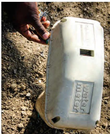
FIGURE 4: A PREPAID METER ON AN INDIVIDUAL DOMESTIC CONNECTION
