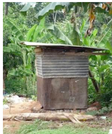
A recently built simple dry pit latrine (Port Moresby)
