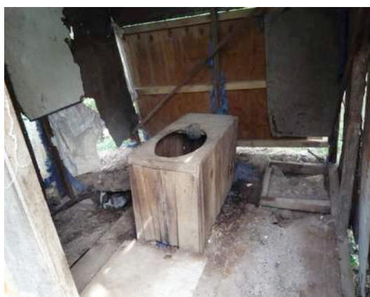
A few toilets were found to have elevated seats, but covering of the pit was rare
