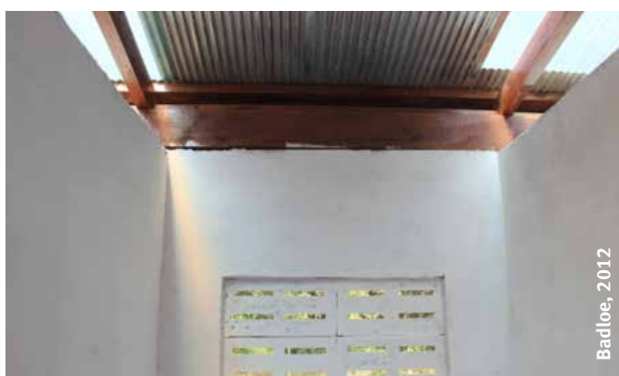
Figure 33: Transparent roof sheets to increase natural lighting
