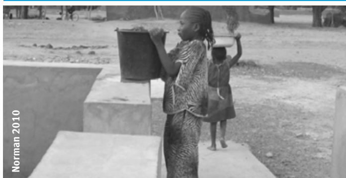
Figure 9: Low enclosure wall can be used as mid-point for resting water container.
