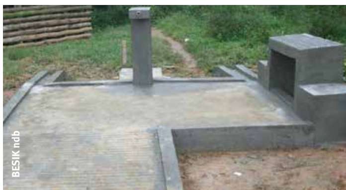
Figure 15: Laundry area at the waterpoint in use.
