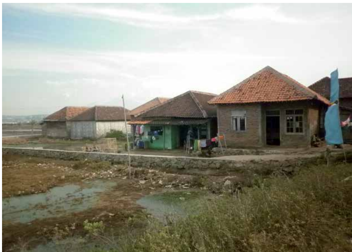
Figure 12. Embankment surrounding houses to protect against flood and sea water inundation in Mangkang Wetan
