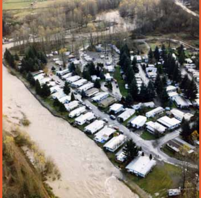
Hazard areas at Riverbend Mobile Home Park
