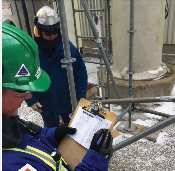
ABM personnel conducting safety assessments and job observation reporting at an ExxonMobil Canada site.
