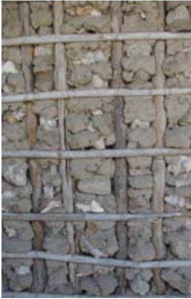
Figure 9 Coral rubble and gastropod shells used in house construction in Northern Mozambique.
