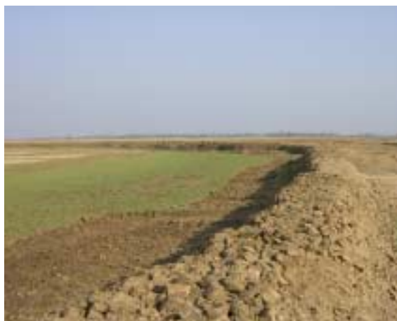
Box 14: Saltwater Embankment
