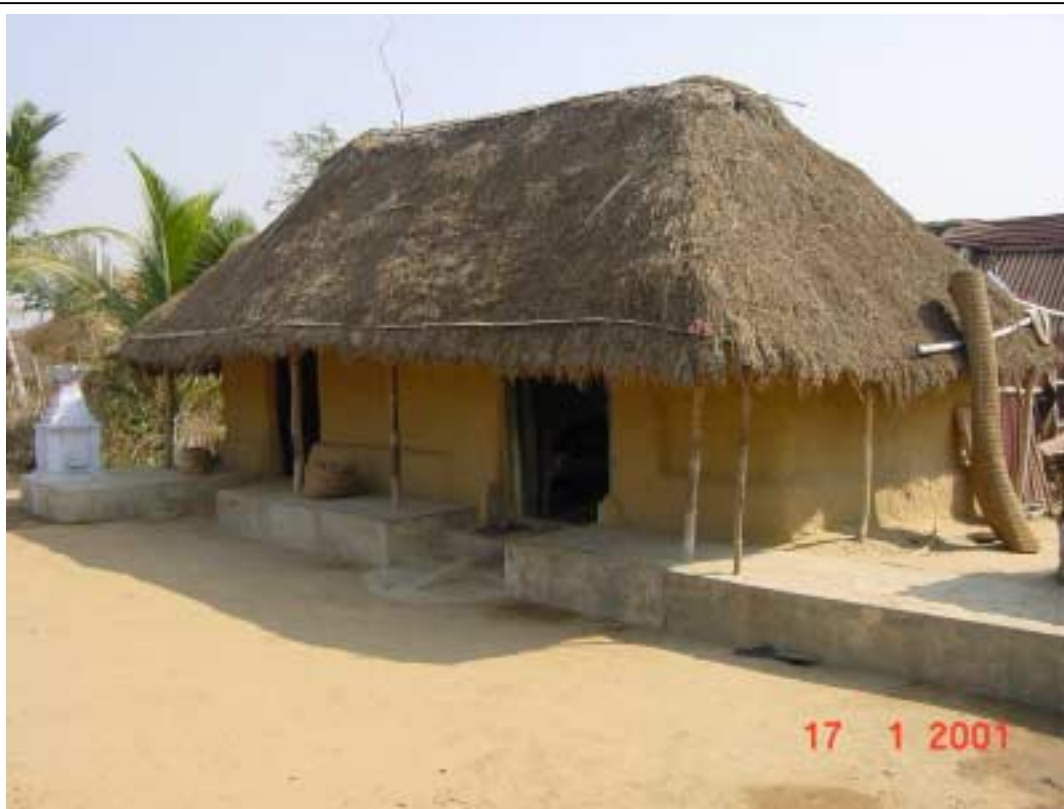
New house constructed under the food for work programme..
