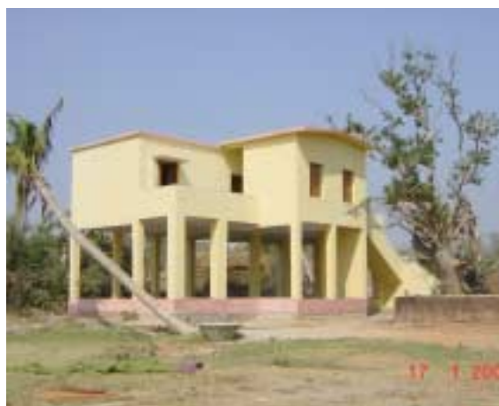
Cyclone shelter built with support from Paradeep Port Trust, in Raskandapur village Jagatsingpur District.
