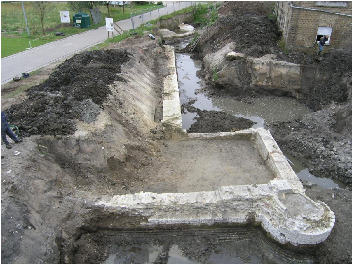
Figure 42 Waterlogged conditions during the excavations of the lower court in 2004.
