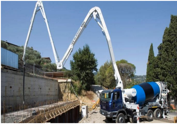
Fig. 3-4: Top-filling process using a truck mounted concrete pump.
