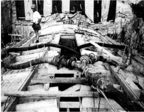
Fig. 3-6: Bifurcated pipeline increasing the rate of placing fresh SCC [3.11].
