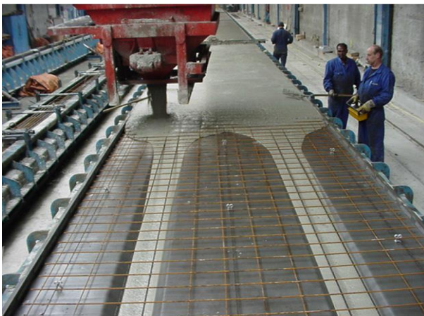
Fig. 3-5: Top-filling process using a skip and a crane [3.10].
