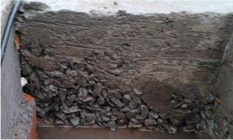
Fig. 2-10: An illustration of segregation of concrete.
