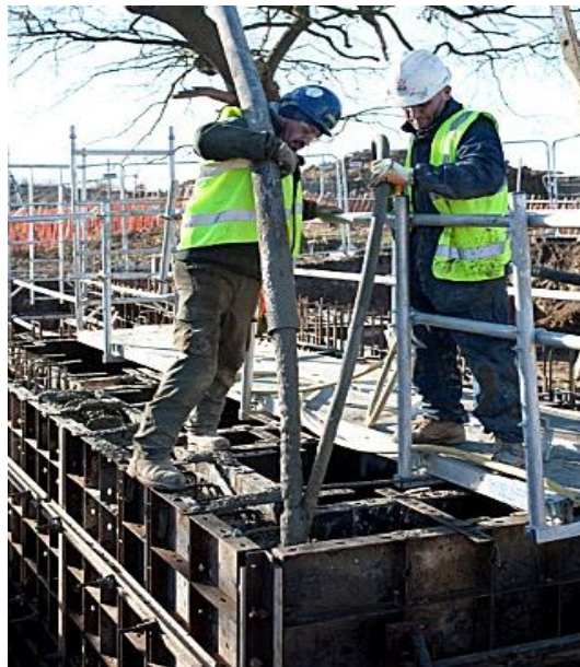
Fig. 3-2: Formwork top-filling process [3.7].
