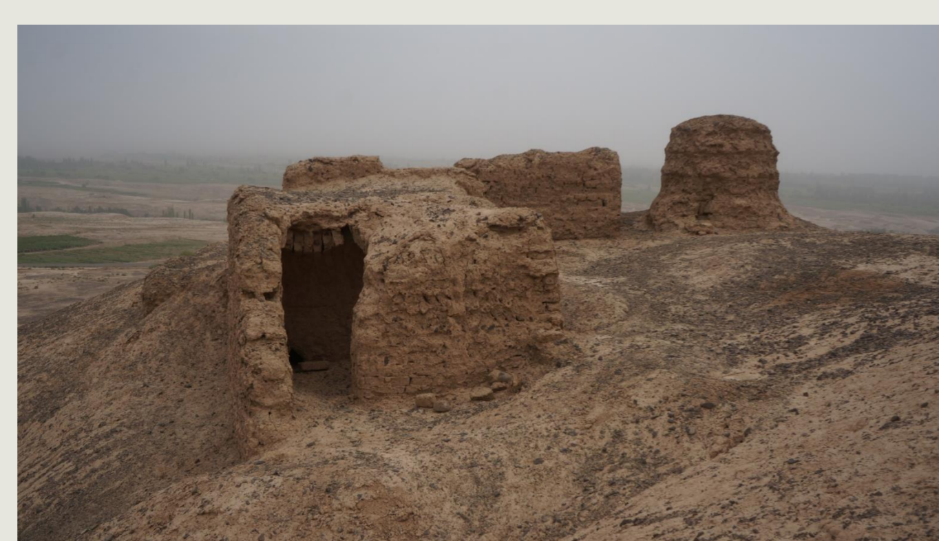
remnants of watch tower
