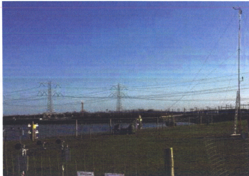
Figure 4 – At the right hand side, a 10m high meteorological mast within the West array location.
