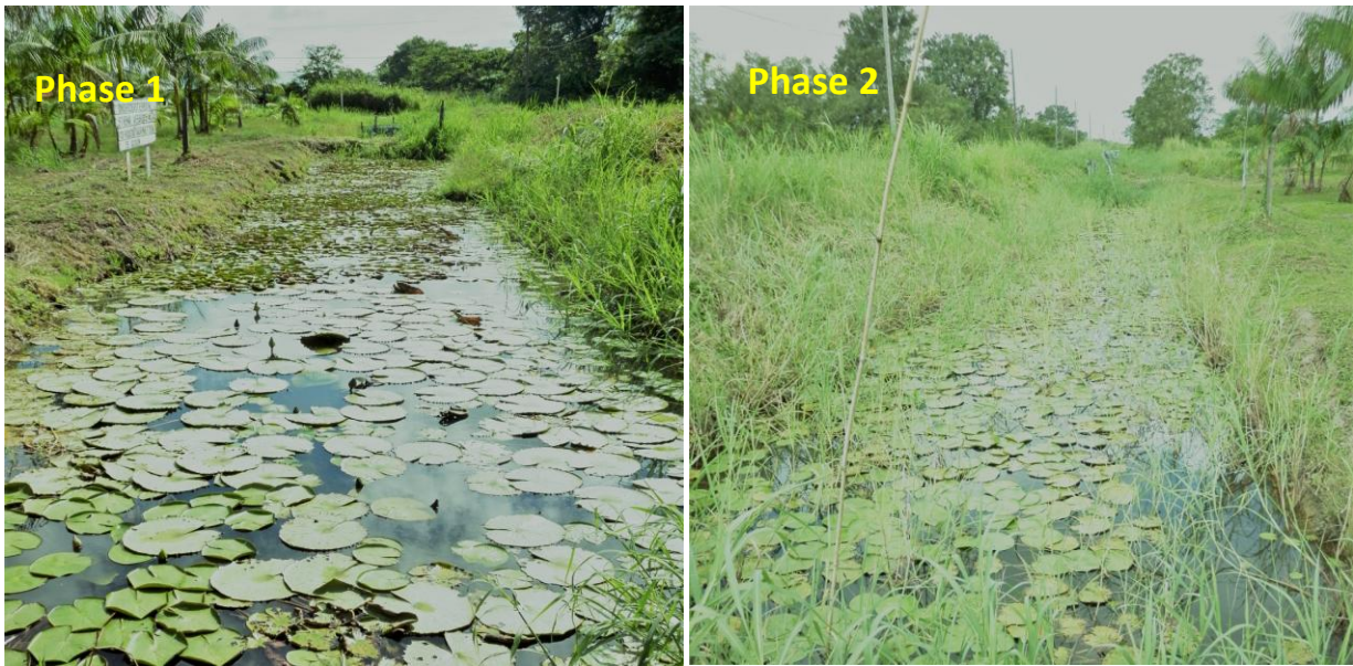
Figure 7-2: Images of the surface flow wetland after the acclimatisation period with Nymphaea amazonum plants (phase 1) and with multiple plant types ( Nymphaea amazonum and Echinochloa polystachya plants (phase 2))
