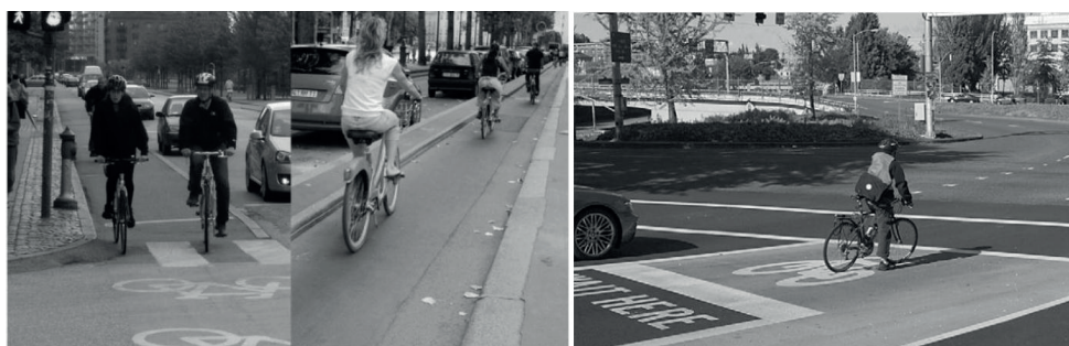
Figure 22. On the left, a bicycle track separated from traffic by a curb. In the middle a bicycle track separated by a parking. On the right, a bike box which is a marked area for bicyclists at intersections (Pucher et al., 2010).
