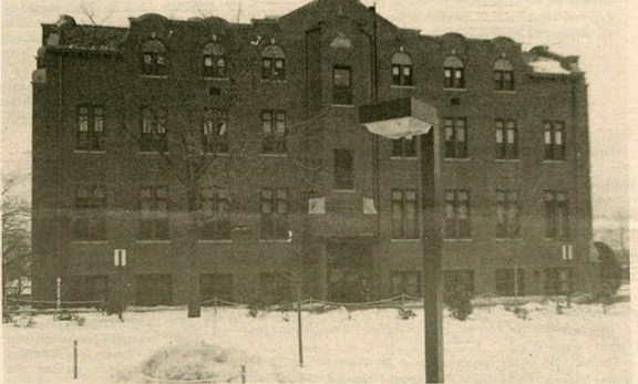
Stephens Hall is one of the numerous buildings containing asbestos on the PC campus which is targeted for asbestos abatement activities. (Photo by Mary Ann Doyle).
