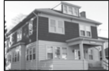
TOLLAMORE 138-140 Radcliffe Avenue
