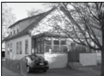
KILLARNEY 93 Pinehurst Avenue
