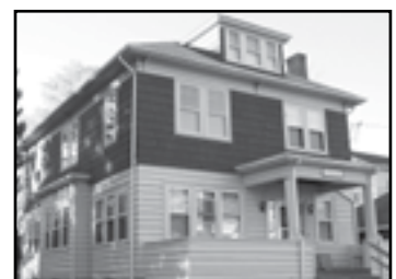
TOLLAMORE 138-140 Radcliffe Avenue
