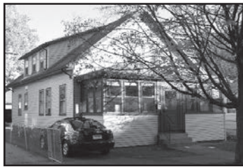
KILLARNEY 93 Pinehurst Avenue
