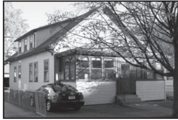
KILLARNEY 93 Pinehurst Avenue
