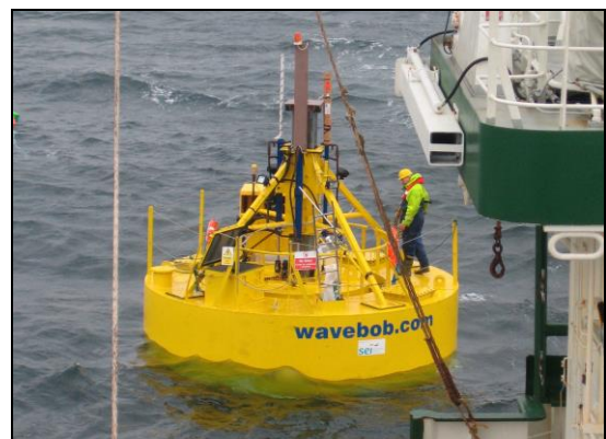
Figure 3. Installation of the Wavebob Device at the Galway Bay Test Site.
