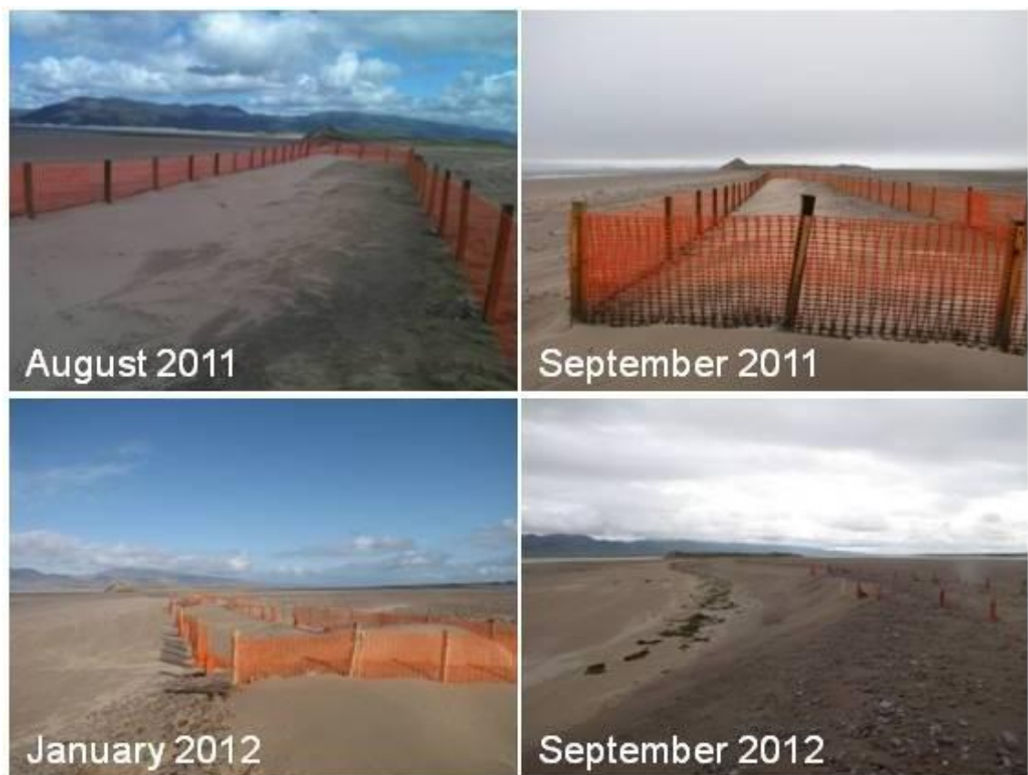
Figure 4.28 Sediment fencing in Location 2
